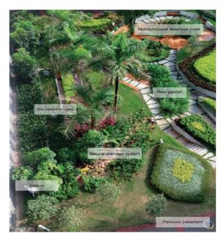
Fig. 2. The LID facilities in the central yard of Civil Engineering Structural Buildings at Shenzhen University.
