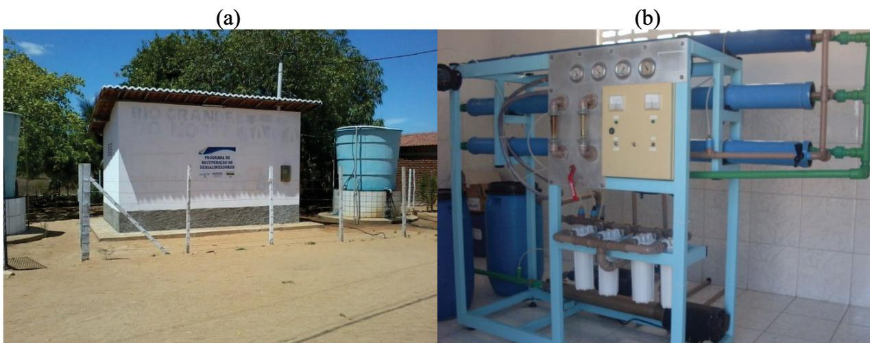
Fig. 1. (a) Desalinator plant and (b) reverse osmosis equipment installed at the communities Alagoinha and Juazeiro in the state of Rio Grande do Norte, Brazil.
