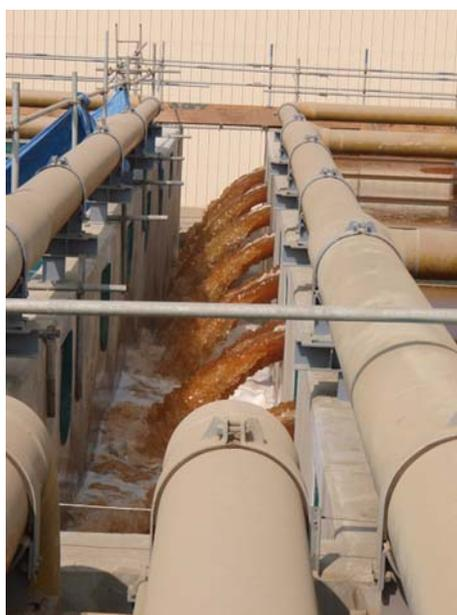
Fig. 1. Picture of the discharge of coagulant ( $\text{FeCl}_3$ ).
