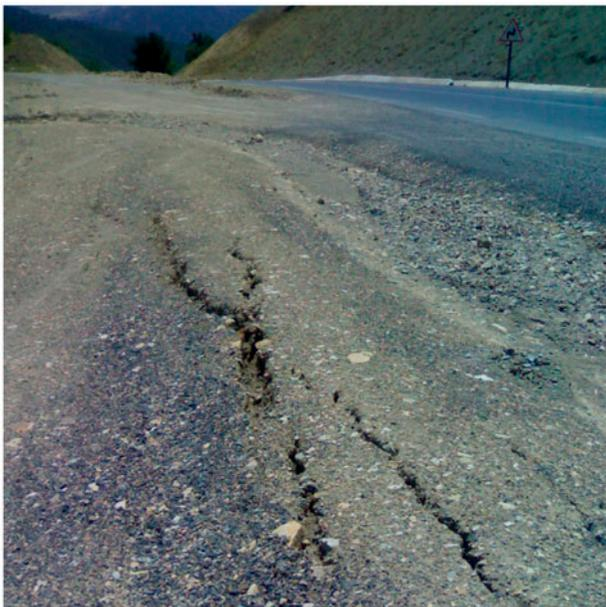
Fig. 1. Cracking of the NR 82 roadway as a result of the argillaceous substratum.
