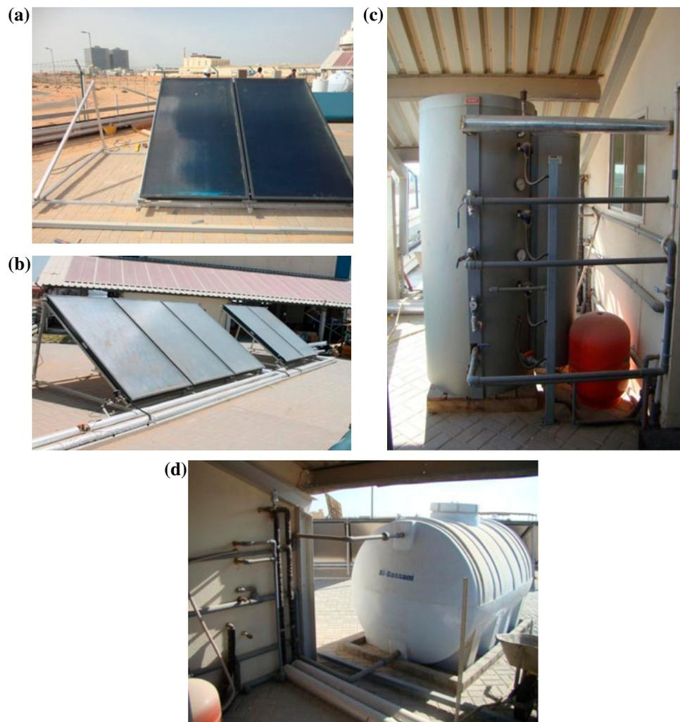
Fig. 5. (a) Installation of flat plate collector plates, (b) orientation, placement and angle orientation of collectors, (c) stratified thermal storage tank with piping circuits, and (d) cold water storage tank (municipal water supply).
