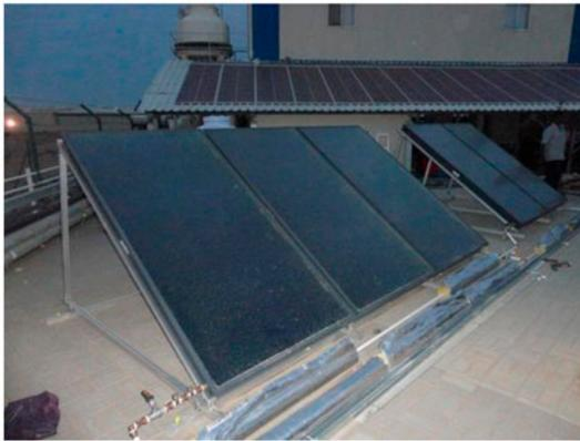
Fig. 8. Flat plate collector array aperture area 11.85 m<sup>2</sup>.
