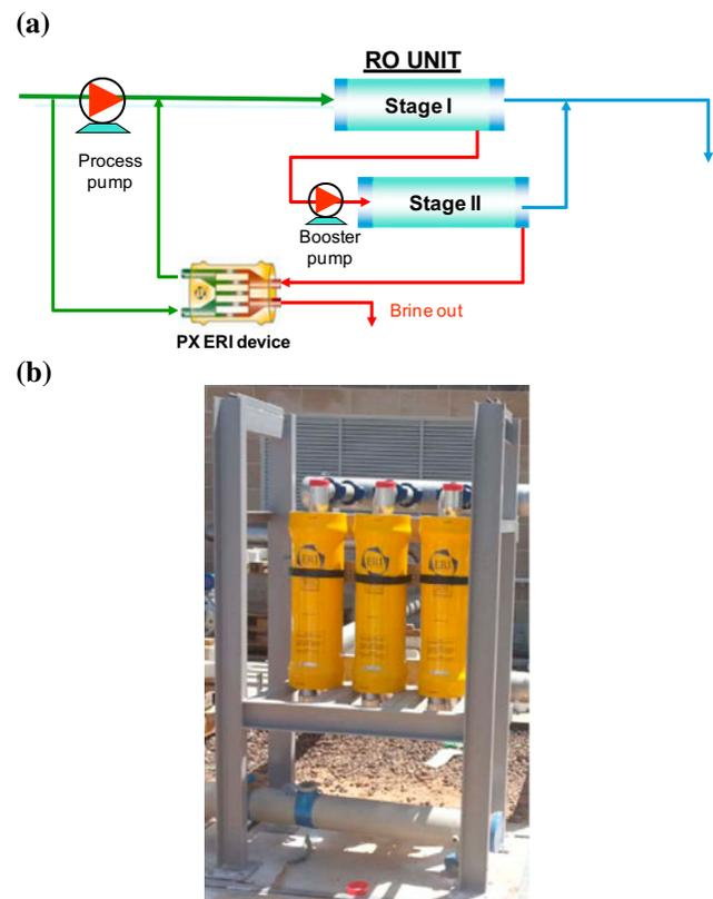
Fig. 9. (a) A schematic illustration of a typical two stage BWRO system with an interstage booster pump and isobaric PX. (b) A photo of one of the PX ERIs in the Lahat 3 and 4 plants during construction.
