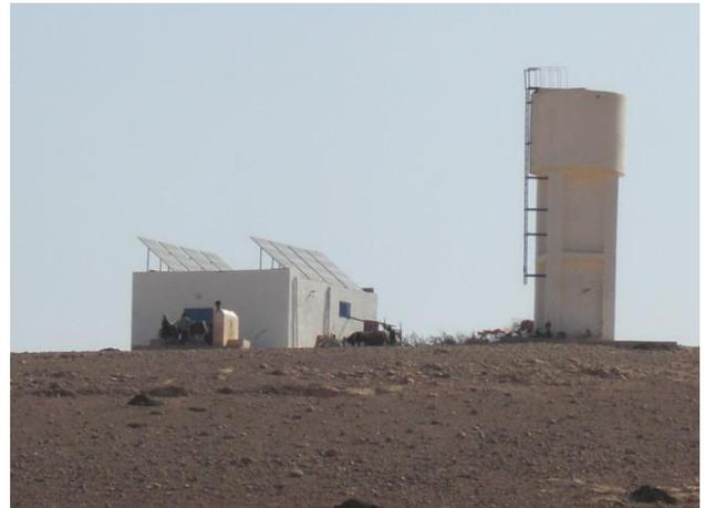
Fig. 30. Fresh water tank, building and PV field (4 kWp) in Morocco.
