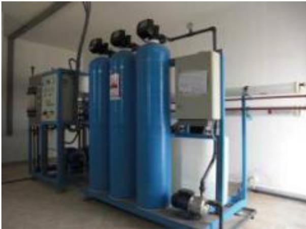
Fig. 29. RO unit installed in Morocco (1,000 l/h)..
