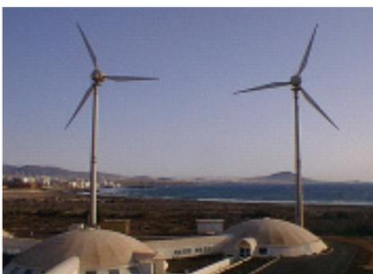
Fig. 5. 2 × 225 kW off-grid wind farm.
