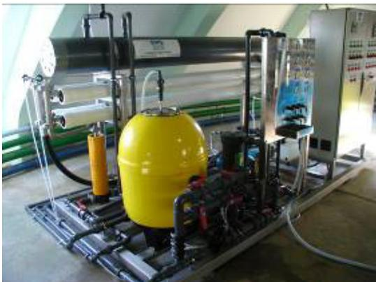
Fig. 23. SWRO desalination plant with ERD (ERI® PX-15).
