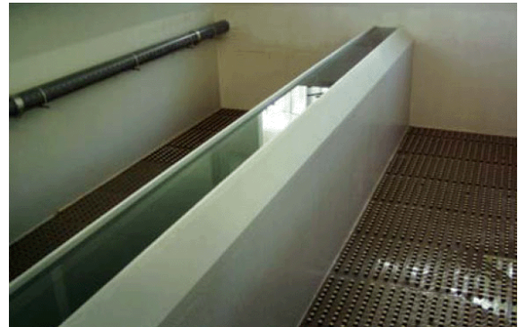
Fig. 8. Eupen calcite filter under construction.
