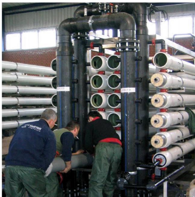
Fig. 3. Typical UF unit with Seaguard membranes.
