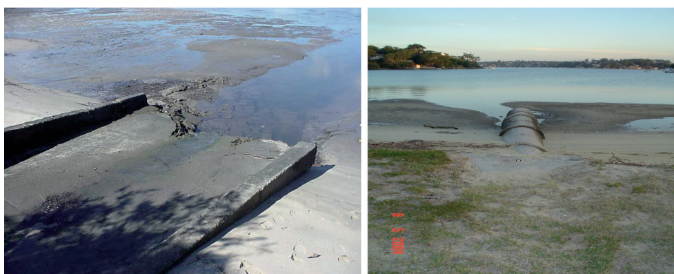
Fig. 1. Sedimentation at connells bay, kogarah.
