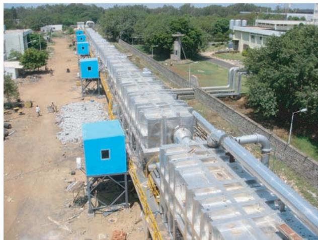
Fig. 1. A view of the MSF module train after thermal insulation.
