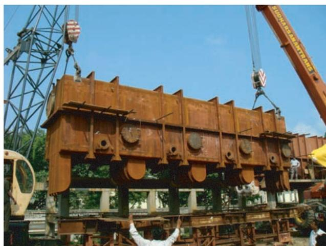
Fig. 15. One of the modules being lifted to mount in position.
