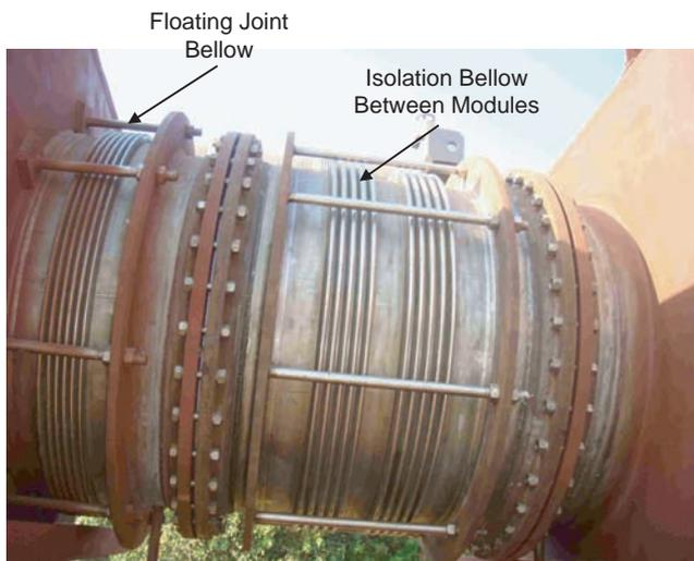
Fig. 8. Typical interconnection between modules for recycle brine.
