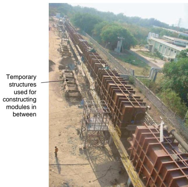
Fig. 14. A view of the module train during construction.
