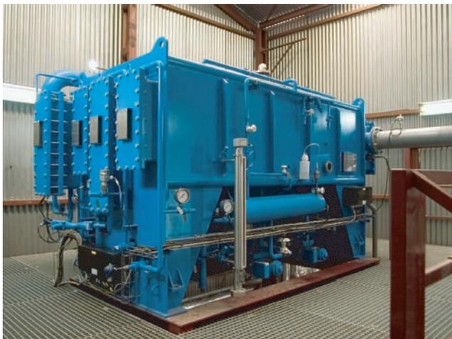
Fig. 1. Double-effect LiBr-H<sub>2</sub>O absorption heat pump in AQUASOL plant.
