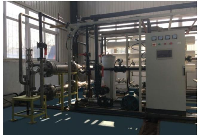
Fig. 4. A photo of the SB-ERD in the SWRO experimental platform.
