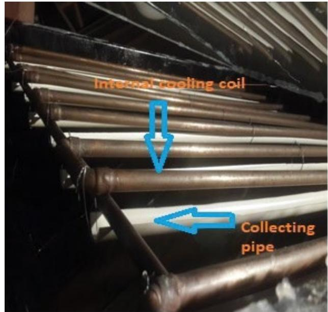
Fig. 3. Collector pipe under the internal coil.
