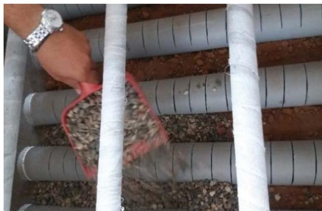
Fig. 1. Clay and gravel placement at the bottom of the biobed.
