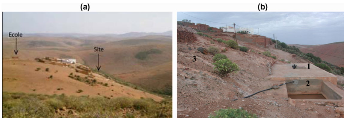
Fig. 1. Site in its initial state. (a) General view and (b) (1) condenser on terrace; (2) double-slope roof condenser and (3) dull condenser on ground.
