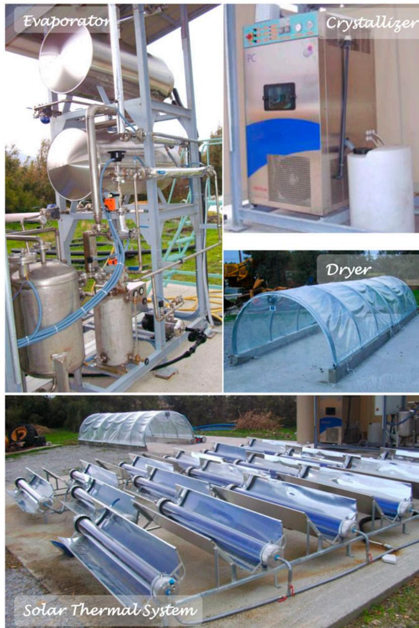
Fig. 9. Photos from the installed SOL-BRINE system.
