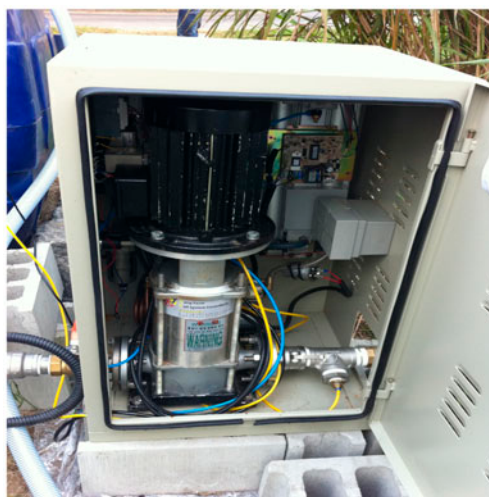
Fig. 1. Micro bubble clarifier.
