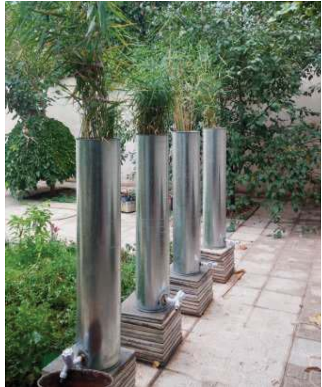
Fig. 3. Vertical flow constructed wetlands during outdoor growth period.
