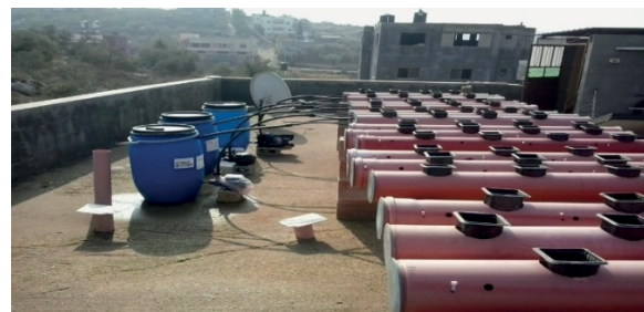
Fig. 3. Picture of the installed hydroponic system.
