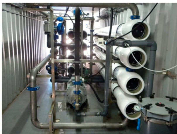
Fig. 4. Closed-circuit seawater RO system.
