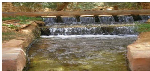
Fig. 11. Small structures composed of dams in the oasis of M'Zab [20].
