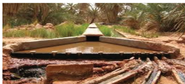
Fig. 13. Foggara water catchment area (Madjen) [21].
