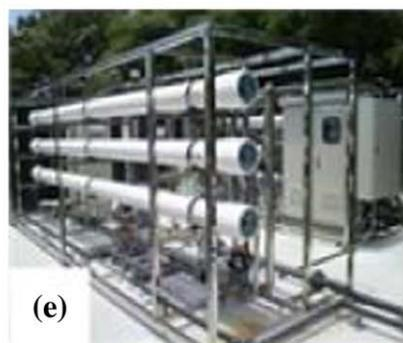
Fig. 3. (a) Schematic drawing of PRO prototype plant, (b) full view of the plant, (c) PRO-unit of the plant, (d) UF-unit of the plant, and (e) low pressure RO-unit.
