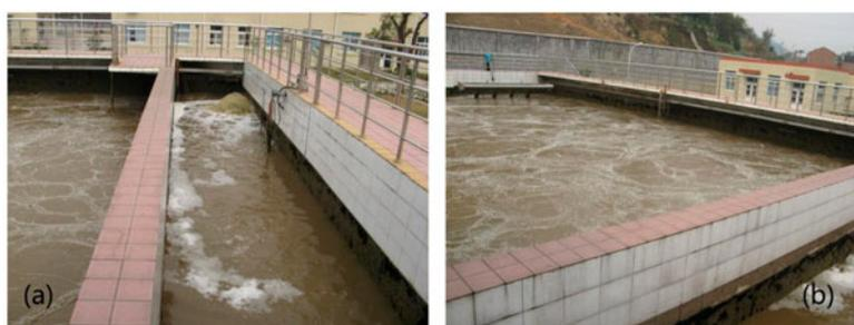
Fig. 2. (a) The biological selection zone and (b) the main reaction area of the CAST biochemical pool.
