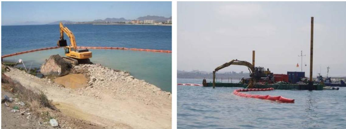
Fig. 8. Turbidity curtain surrounding the dike and barrier construction (left) and the marine excavation works (right).
