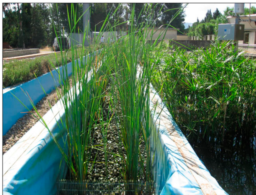
Fig. 1. A view of pilot-scale HSSF system located downhill from the sewage plant in Piana degli Albanesi (Sicily, Italy).
