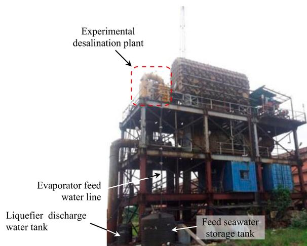
Fig. 3. Pictorial view of the desalination plant installed in the power plant.
