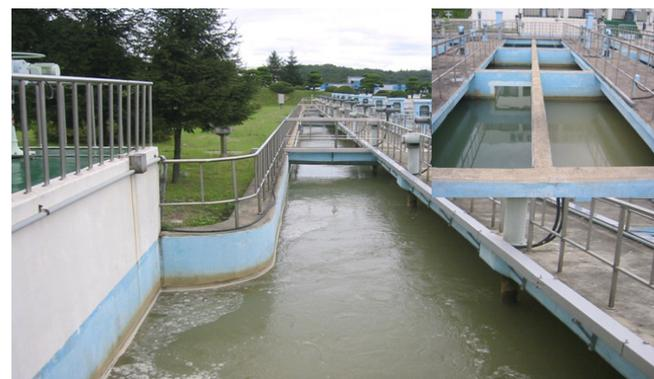
Fig. 4. Actual distribution channel and flocculation basins in S\_WTP.
