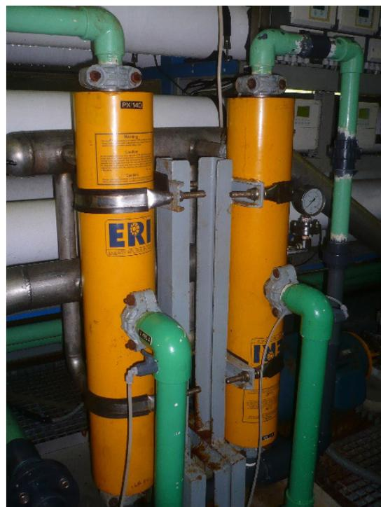
Fig. 2. Energy recovery device.
