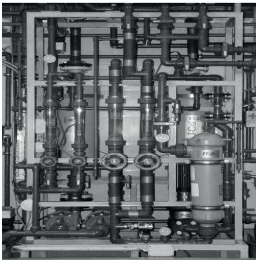
Fig. 2. Liqui-Cel™ Membrane Contactors with operation panel at Budapest's TMCS plant.
