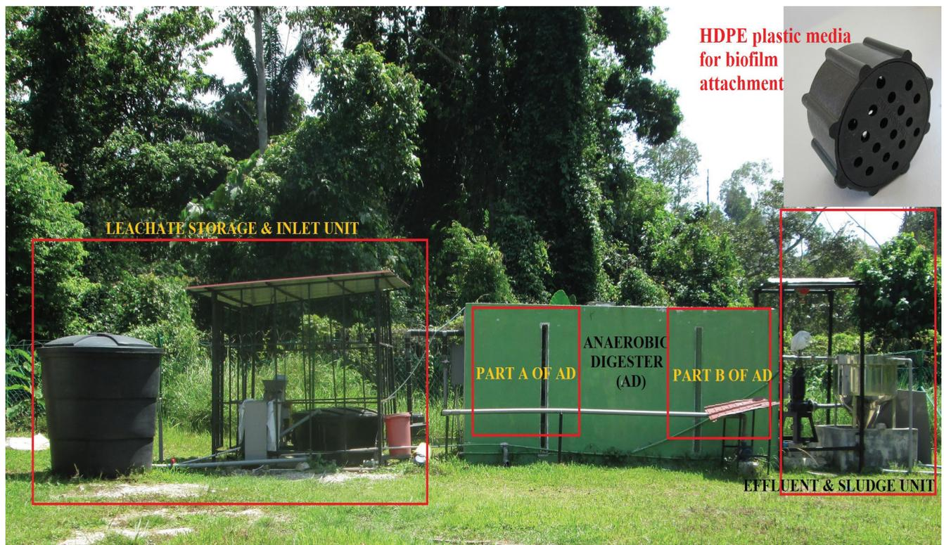
Fig. 2. Pilot-scale ABD system at UKM biogas site.
