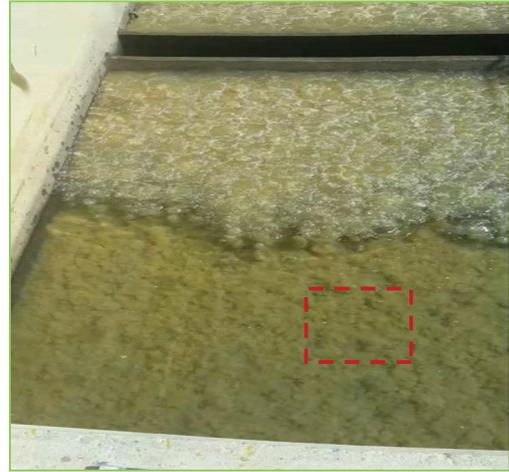
Fig. 3c. Algae accumulation on the filter surface at 2 pm.
