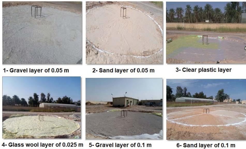
Fig. 5. Different steps for preparing the collector ground.
