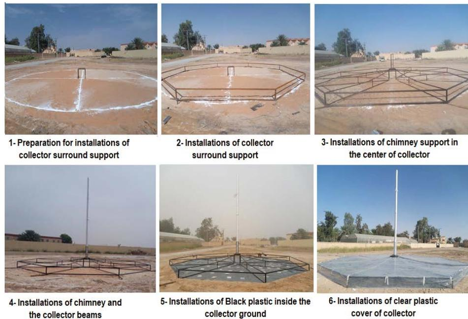
Fig. 6. Different steps for the construction of the collector roof.
