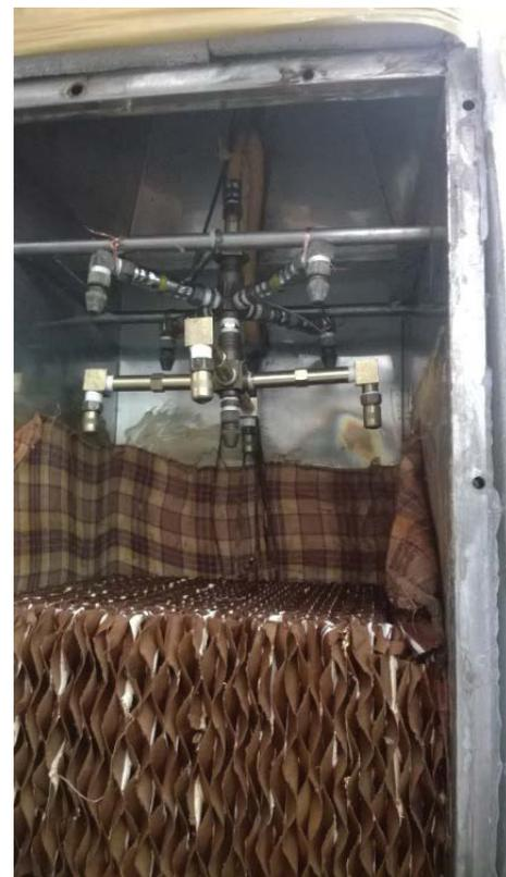
Fig. A2. Inside space of the humidifier presented in Fig. 4.
