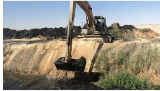
Fig. 11. Dredging operation of Oued Righ channel.
